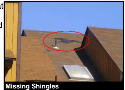
Missing Shingles
